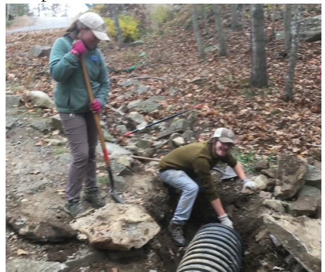
Below: Trail Crew installing a new culvert on Hairpin Trail.
